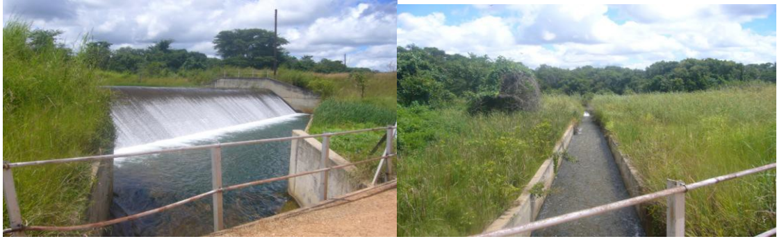
Figure 6: Photos showing spillway and main canal
