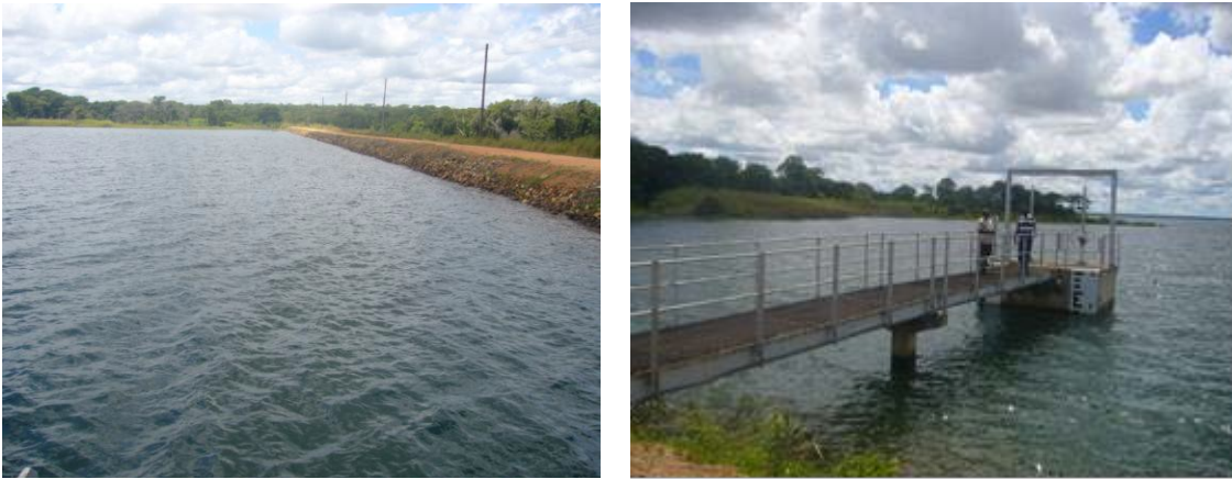
Figure 9: Photos showing the dam, platform for gauging, spill-way and open canal
