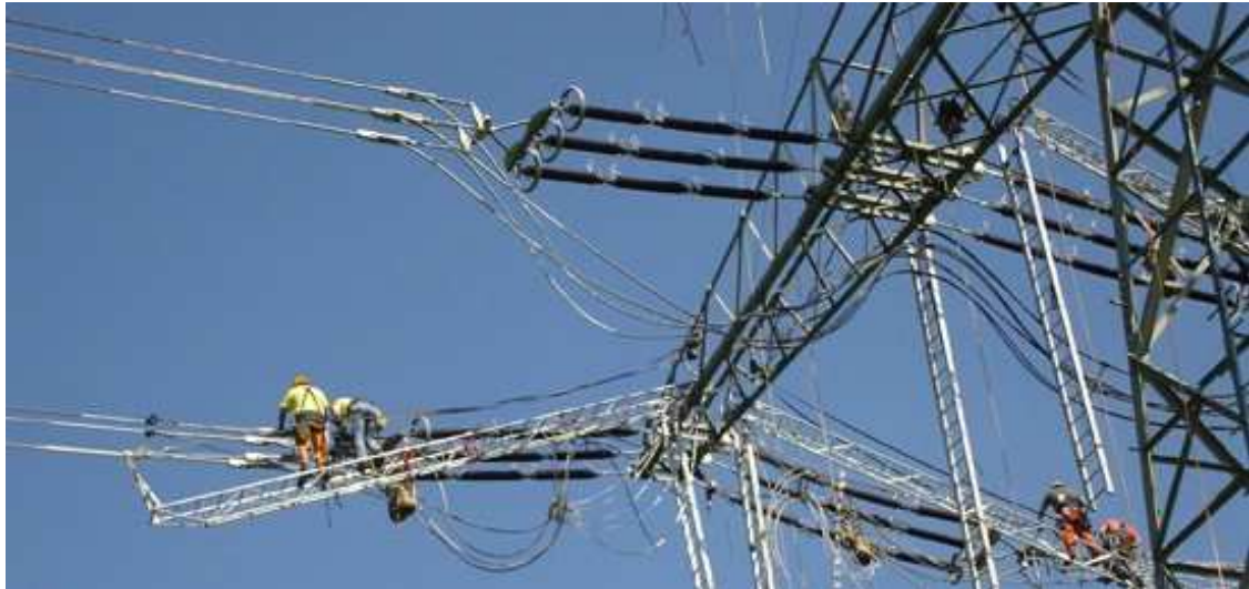
Figure 3.12: Strain Tower, Clamping 3 Bundle Conductors - Jumper Loops Unfinished
