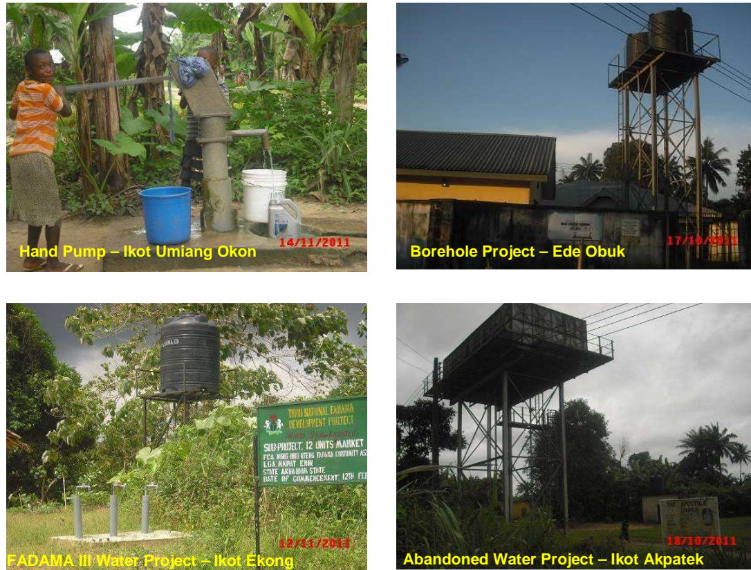
Figure 4.39: Water Supply Facilities
