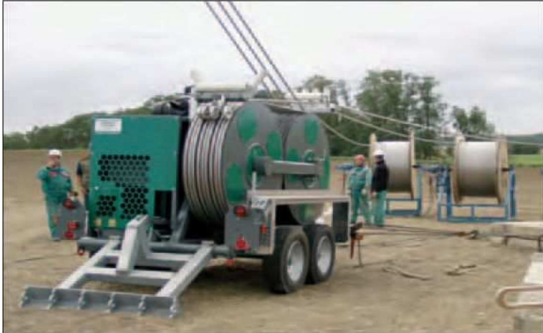
Figure 3.11: Puller- Tensioner during Stringing of 3 Bundle Conductors
