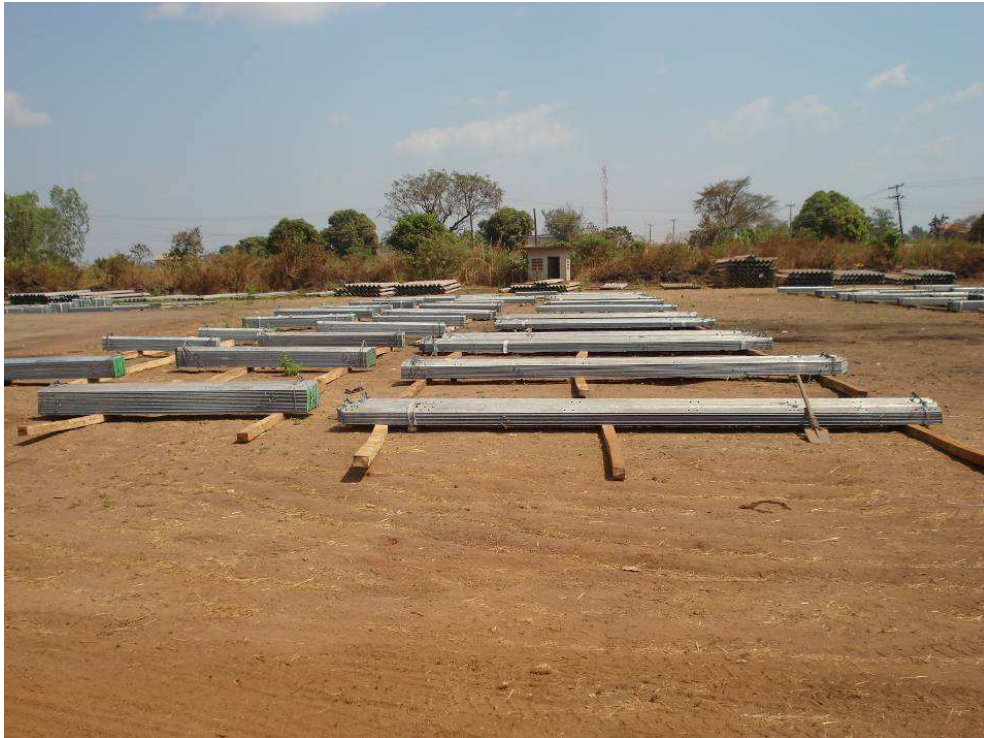
Figure 3.5: Lay-down Tower Materials Storage
