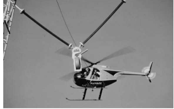
Figure 3.9: Helicopter Pulling a Pilot Wire
