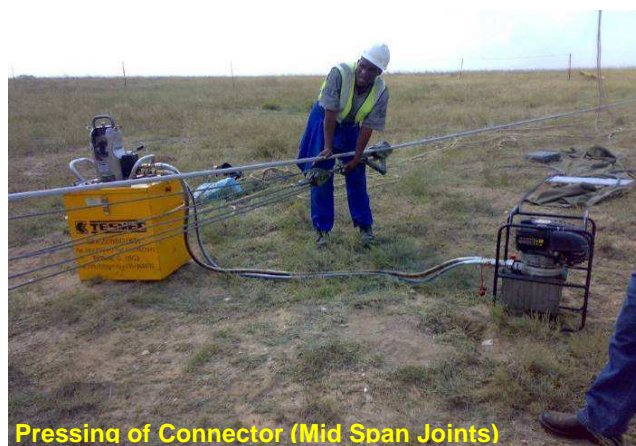
Figure 3.2: Typical Connectors Pressing
