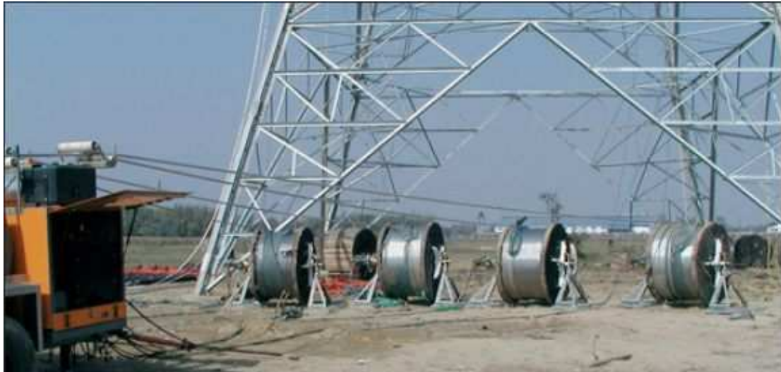
Figure 3.10: Drum- Stand with Hydraulic Drive and Disc Break
