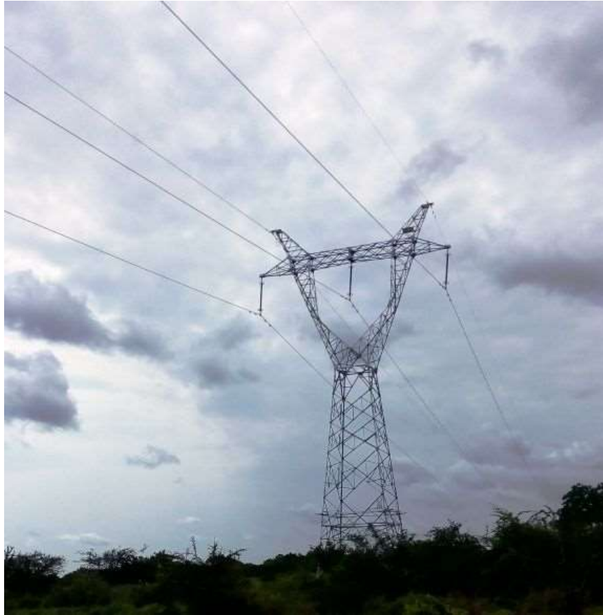
Plate 6: High Voltage Electricity line cross cutting the project site
