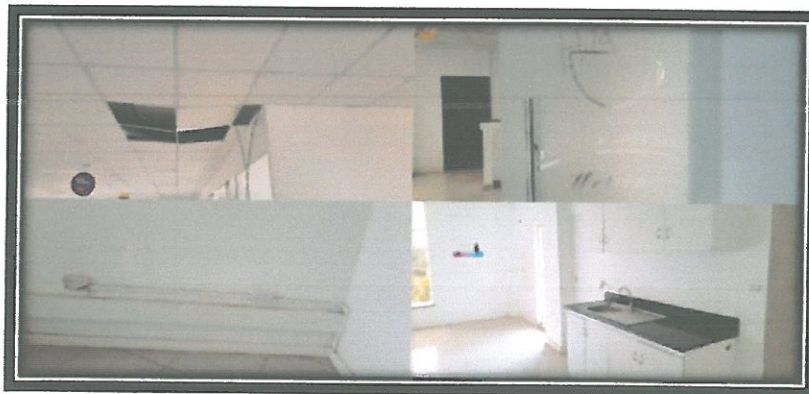
Figure 2: Office rooms to be refurbish
