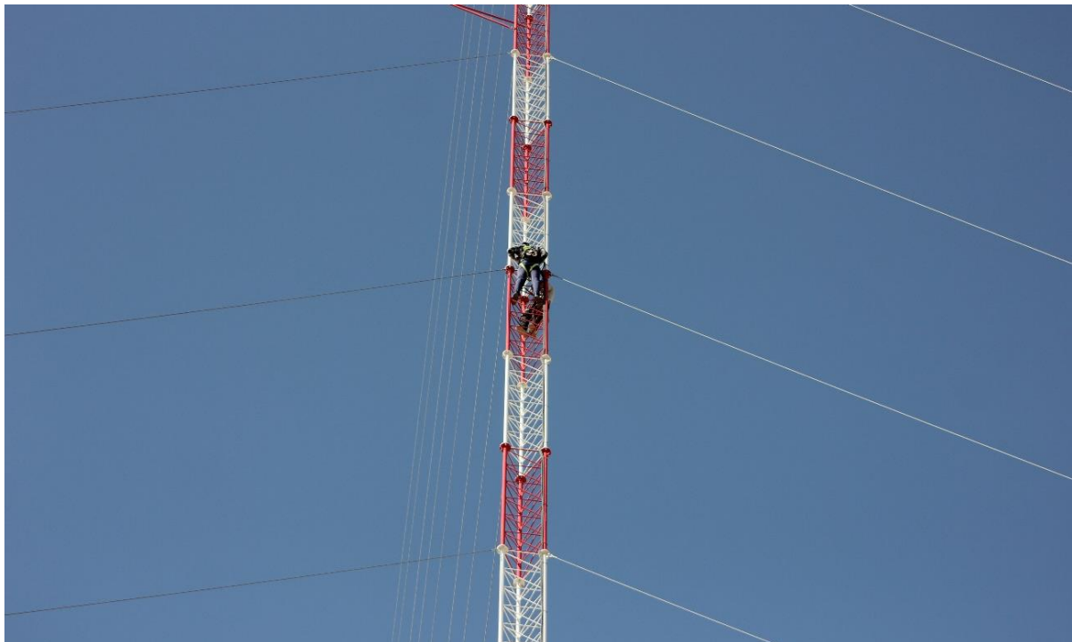
Figure 4-2 Bat detector installation on weather mast in Bash project area
