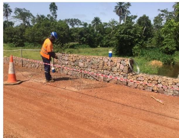
Figure 9: Construction des gabions
