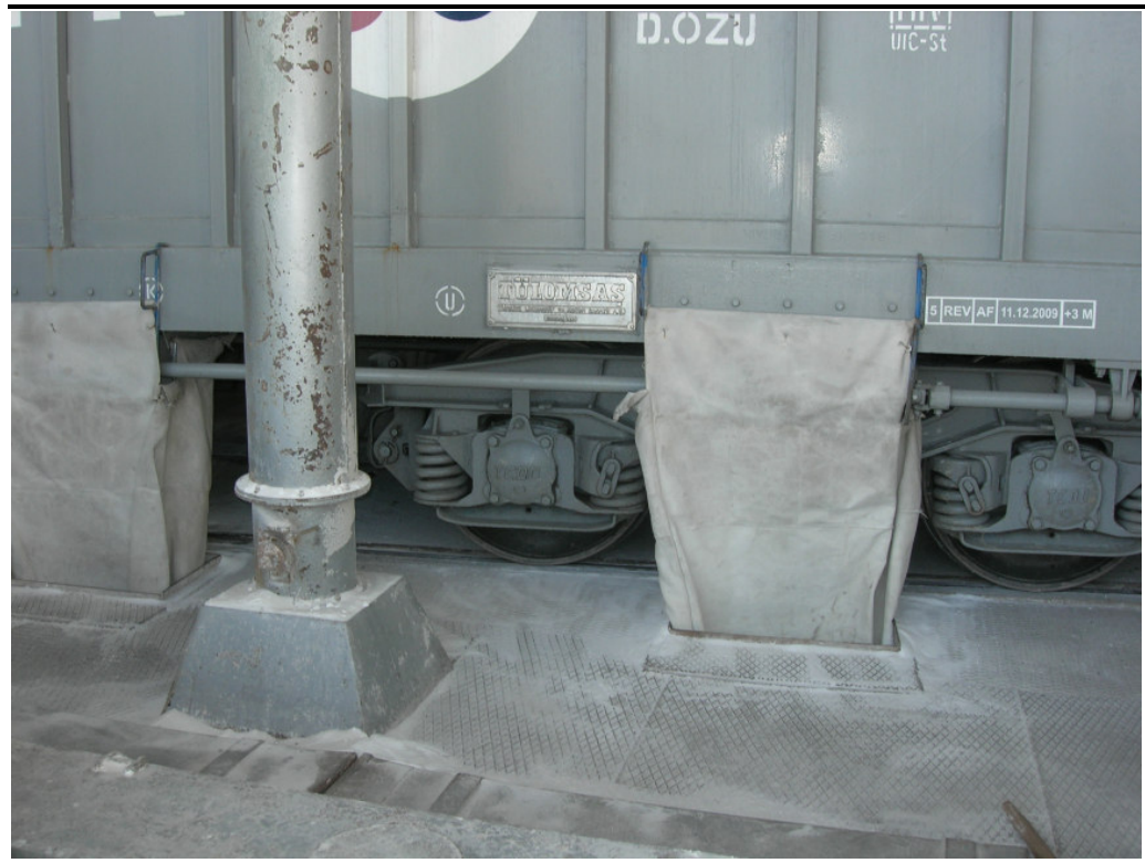
Box 1.15 ETI - Dust Suppression
