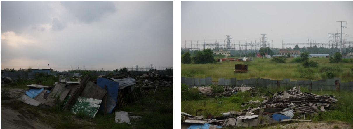
Wastes from demolished labor sheds
