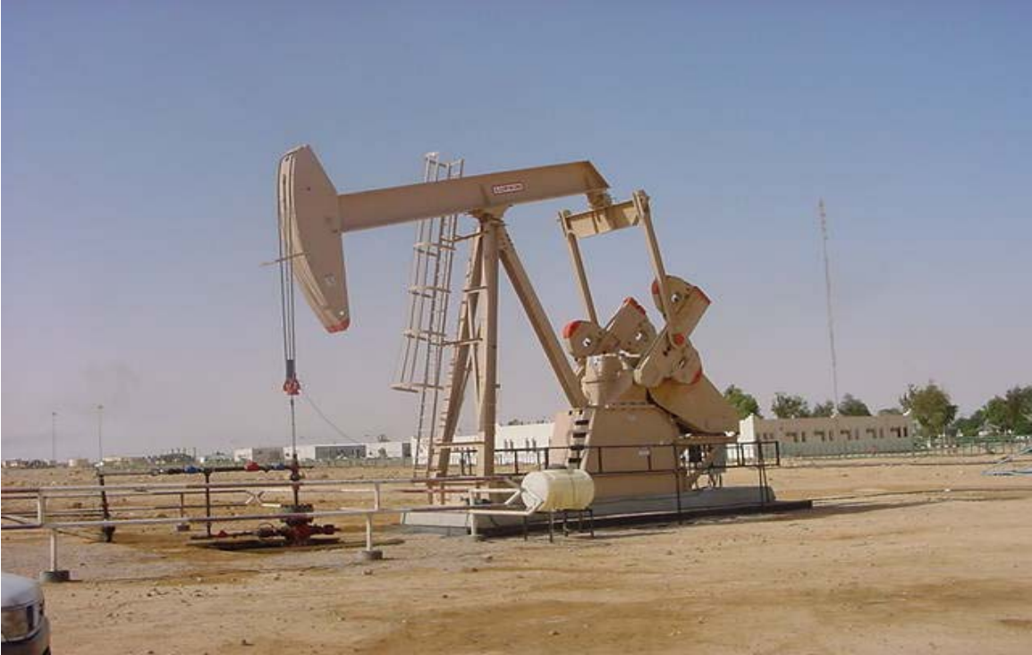
Typical Oil Well – With Pump-Jack (Khalda)
