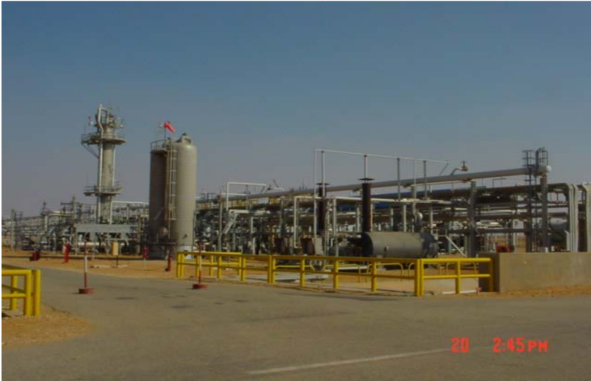
Qarun Oil Process Facility
