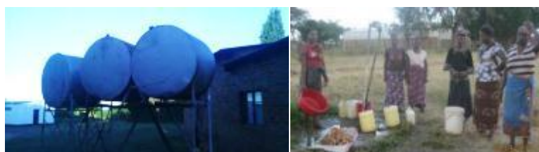
Figure 22: Borehole Water Reserve Tanks and Water collection points at the Farm
