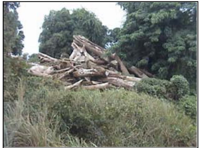
Photo 3-5 DUEY RIVER BED AND CHARACTERISTICS OF ITS BANKS
